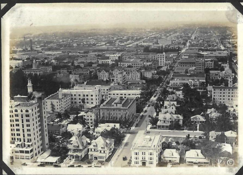
THE HEART OF MIAMI LOOKING WEST ON ELEVENTH STREET.
